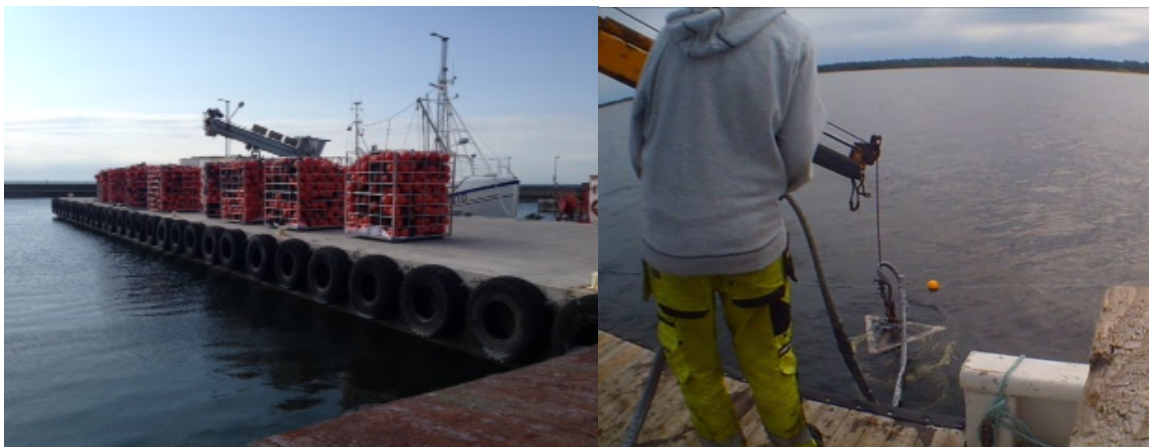
Figure 14. Left: The net farm in Byxelkrok arrived to the quay in pre-made units. Right: Drilling anchors into the sea-floor is time-consuming compared to other anchoring methods.
